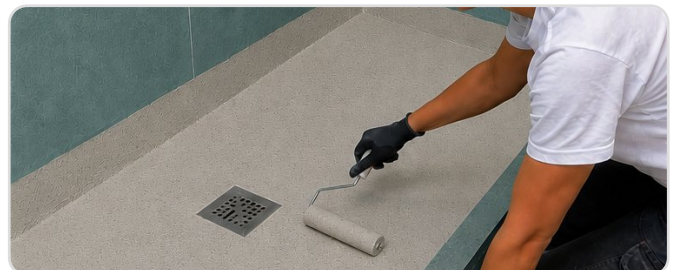
Shower tray waterproofing
