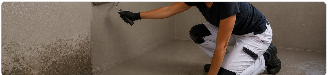
Damp-proofing treatment of a basement wall and floor slab with IMPERFLEX FIBER-1C
