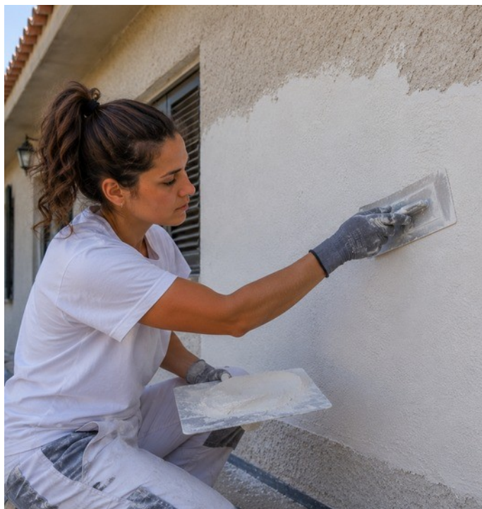
Levelling a façade with TECNOCEM COSMETIC
