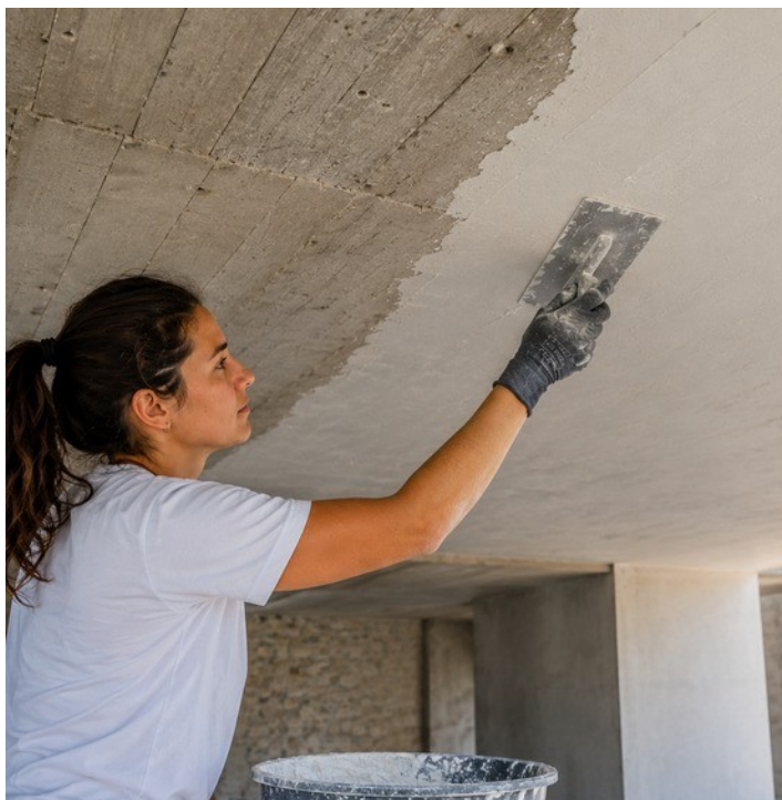
Smoothing a concrete ceiling surface
