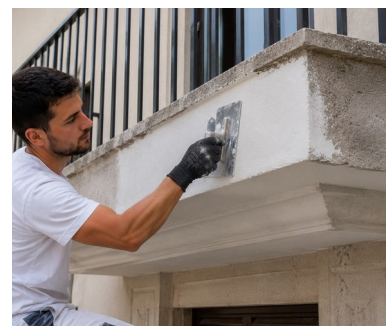
Repairing and smoothing a balcony edge with TECNOCEM COSMETIC
