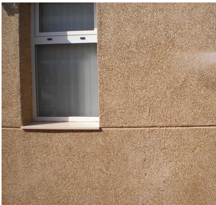
Hidro-A applied to a single-coat render façade
