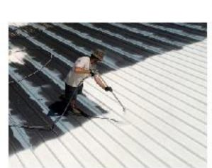
To achieve an optimal result in terms of thermal insulation, it is recommended to apply 3 layers, the 1st diluted in 5% water and the remaining two pure or with a maximum of 5% water,
